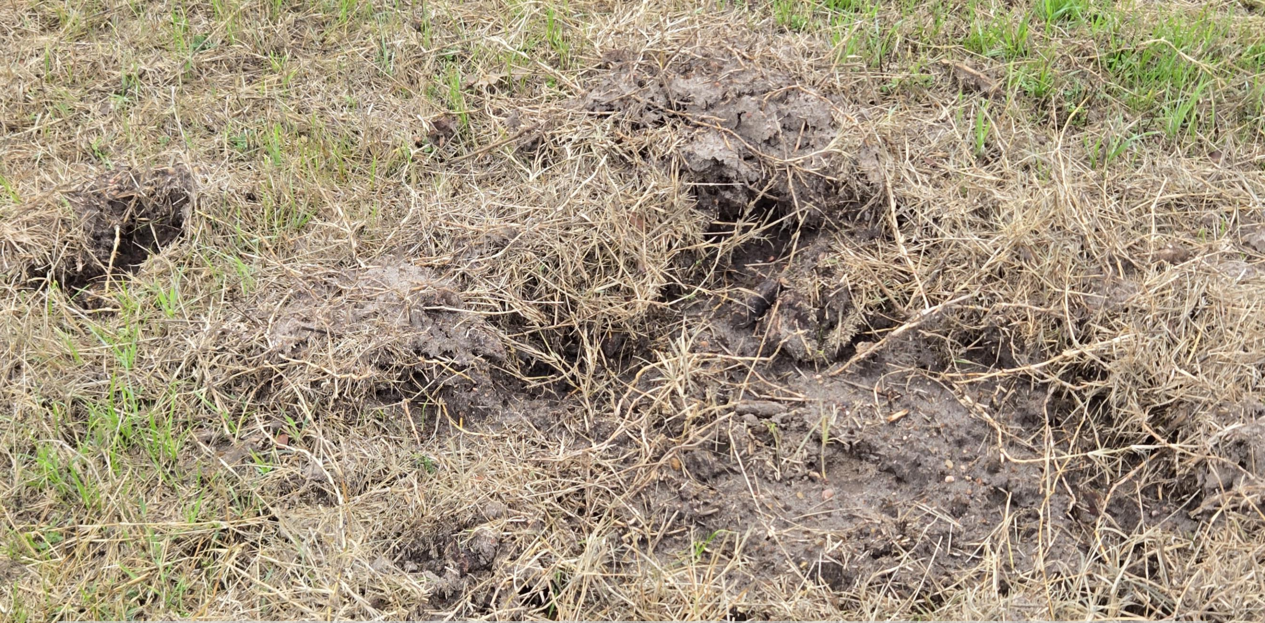
Feral Hog Damage on Levee of the Primary Emergency Spillway
